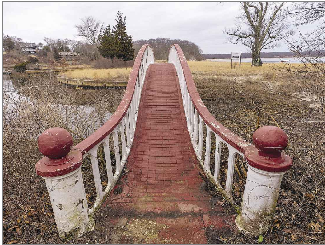
The rebar-concrete Ransome Japanese Bridge was named to the National Register of Historic Places.
