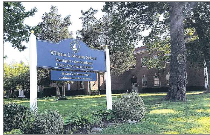
The administrative offices of the Northport-East Northport School District on Laurel Avenue in Northport.
