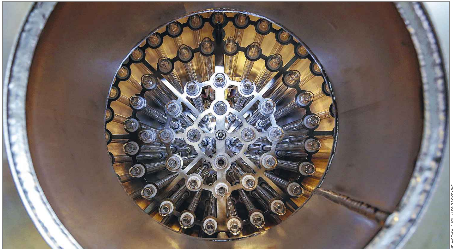
The Suffolk County Water Authority ran a pilot test, using ultraviolet lamps, above, in its ultraviolet reactor at its pump station in Central Islip.
